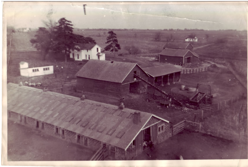
The Agnew farm as it looked when the folks bought it in the late 40s. Most of the buildings visible in this photograph are now gone.
